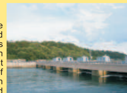
The tidal power station in the Rance river, France, built in 1967.
