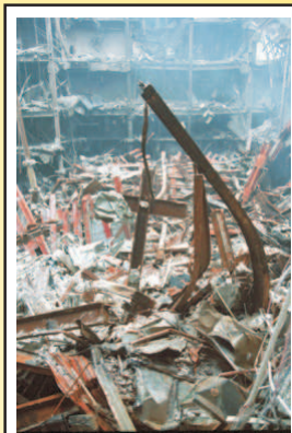
Twisted girders and rubble after September 11th.
